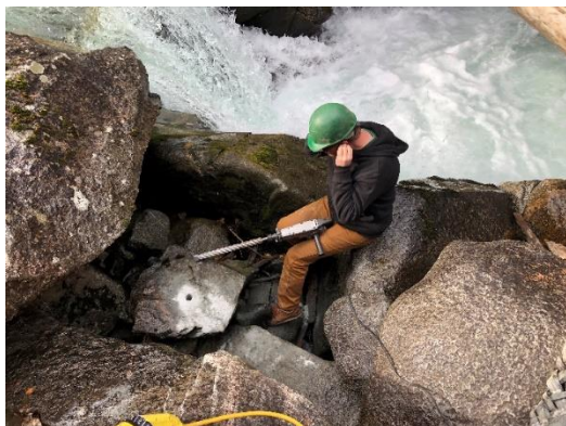
Dry pit below the Lostine River Falls before modifications
