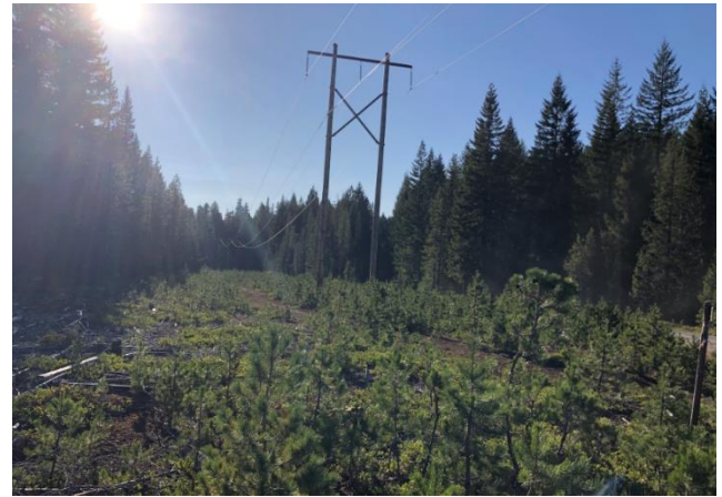
Potential wildlife habitat under powerlines
